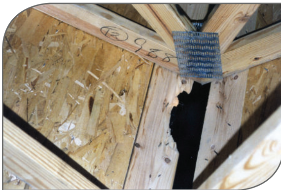
Examples of improper ridge vent openings
