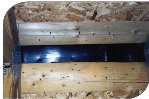
Examples of improper ridge vent openings
